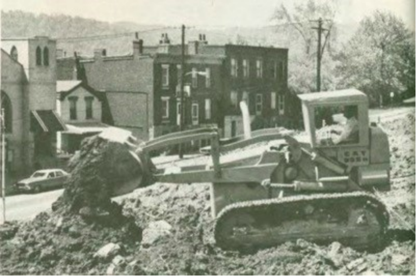
Image 7 - Bulldozers on Chapline Street, 1971. 48
