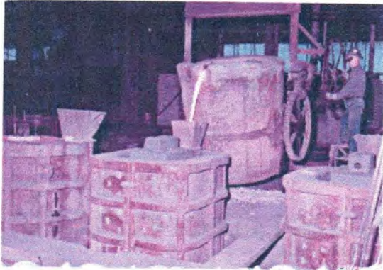
Pouring iron from ladle into molds.
