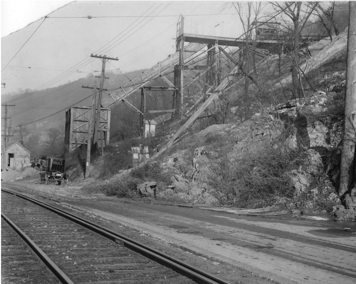
Tipple, Richland/Costanzo coal mine, South Warwood, circa 1914-20.
