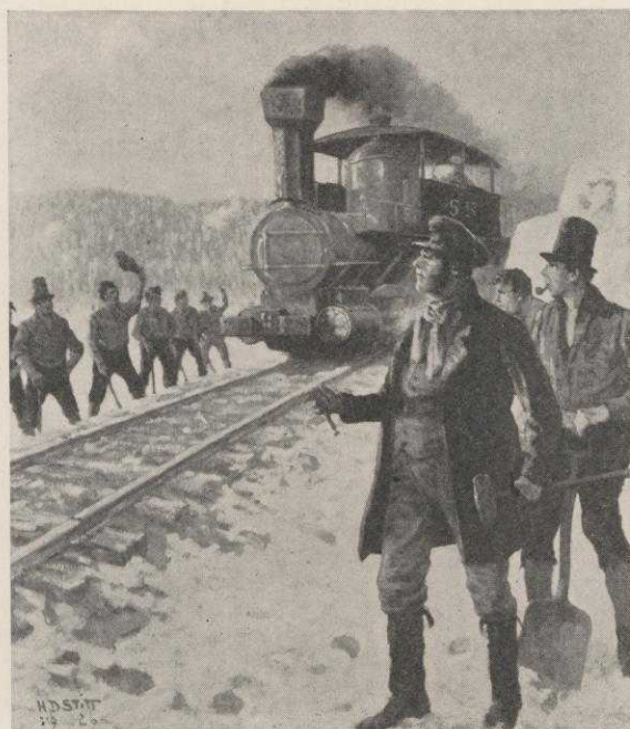
ROSEBY'S ROCKS, December 24, 1852 The last spike is driven, completing the B. & O. to Wheeling. This picture is from a painting which will be part of the B. & O. display during Centennial Week.
